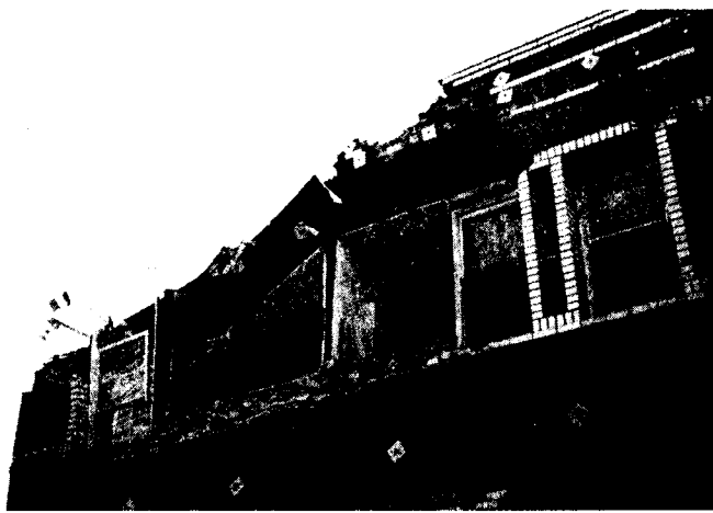
FIG. 2. Failure of URM Wall That Was Retrofitted by Tying Floor Beams to Wall
