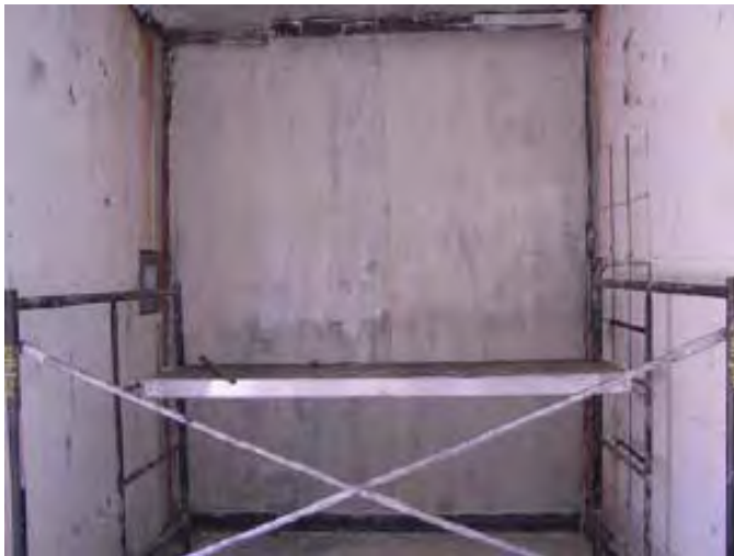
Figure 3. Interior view of retrofitted wall
