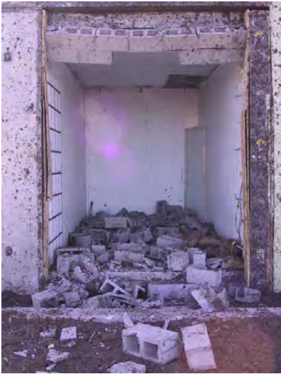
Figure 7. Post-Test view of control wall
