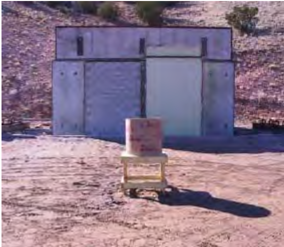
Figure 5. Exterior view of test structure and explosive
