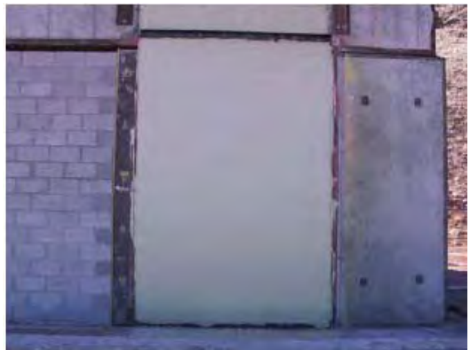
Figure 4. Exterior view of retrofitted wall
