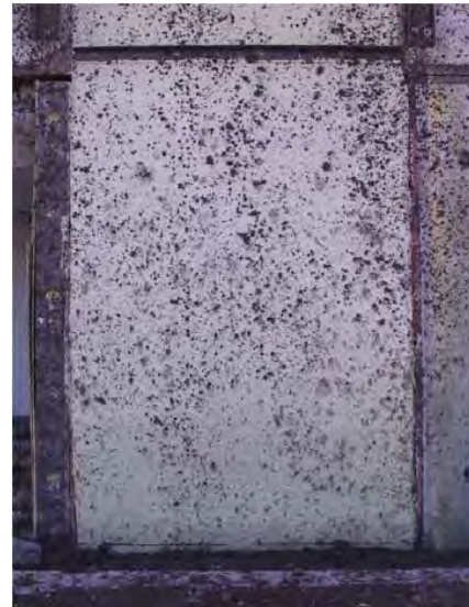
Figure 8. Post-Test view of retrofitted wall
