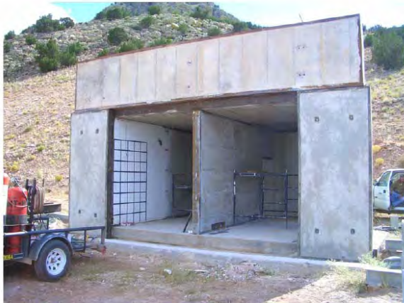
Figure 1. Containment Structure before installation of CMU walls
