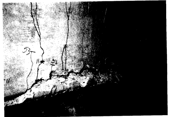
Fig. 2—Local failure in reinforced concrete beams strengthened with FRP plates
