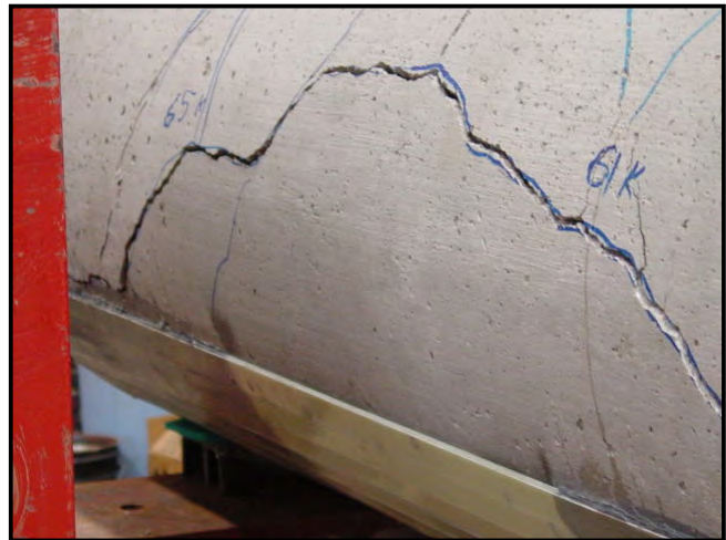
Figure 15. Enlarged shear crack in Specimen 3, Test 3.
