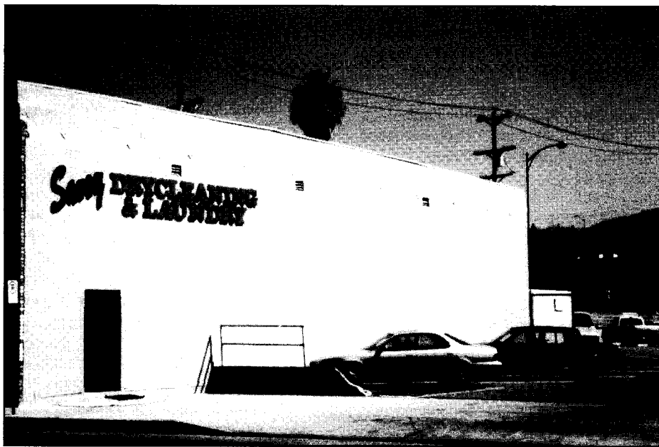
Fig. 14—Exterior of wall at completion of project (Photo courtesy of External Reinforcement, Inc.)
