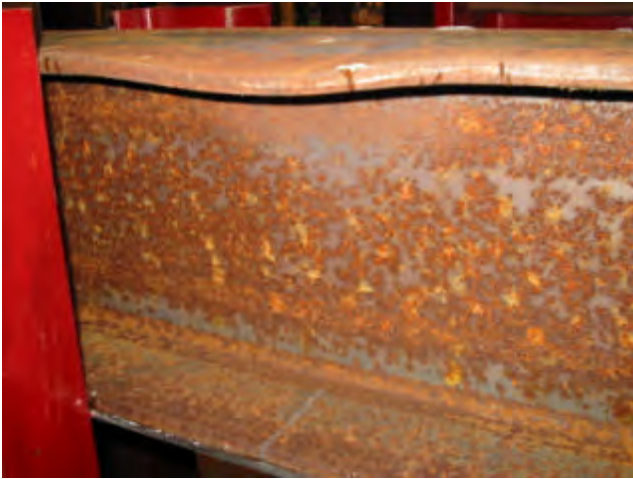
Figure 6. Local deformation of compression flange under point of applied load.
