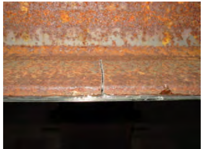
Figure 2. Tension flange cut on both sides of web.
