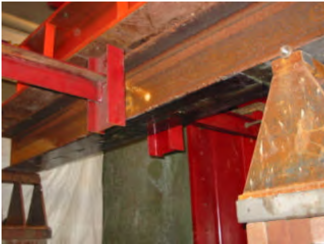
Figure 3. Carbon laminates on tension flange.
