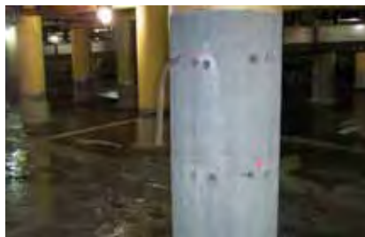
The repair method developed by HJ3 Composite Technologies involved (top to bottom): removing damaged concrete from columns and patching damaged areas with polymer material resistant to chemicals of pH 1 or less; installing vertical fiber-reinforced polymer (FRP) strips; and wrapping with FRP fabric.
