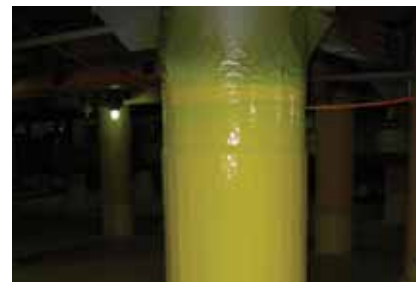
The repair method developed by HJ3 Composite Technologies involved (top to bottom): removing damaged concrete from columns and patching damaged areas with polymer material resistant to chemicals of pH 1 or less; installing vertical fiber-reinforced polymer (FRP) strips; and wrapping with FRP fabric.
