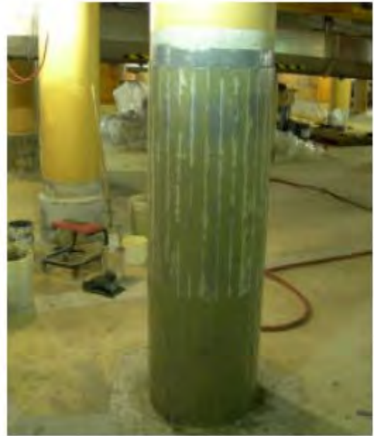
Pic 8: HJ3 System Installed
